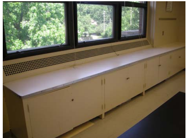
Fin Tube Enclosure and Casework
