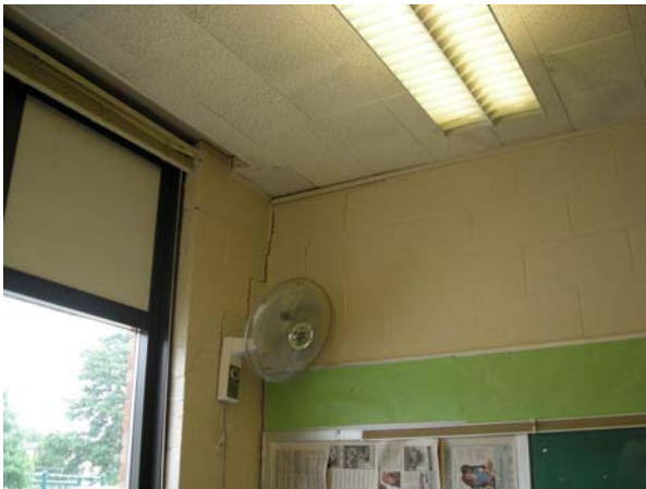
Cracking in CMU partition wall
