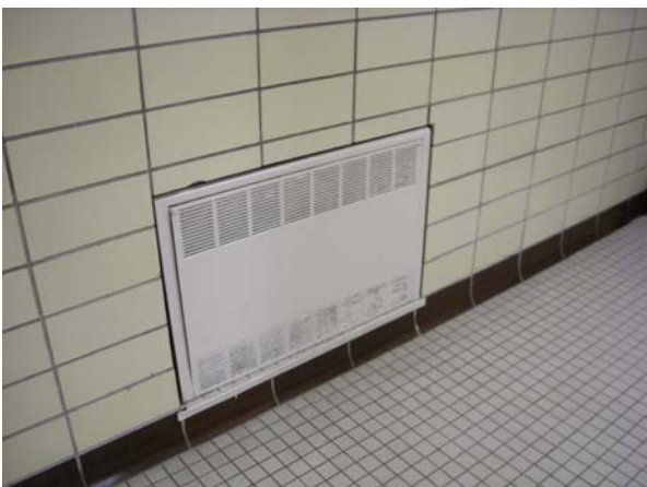
Unit Ventilation in Restroom
