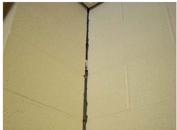
Separation of partition wall from exterior wall
