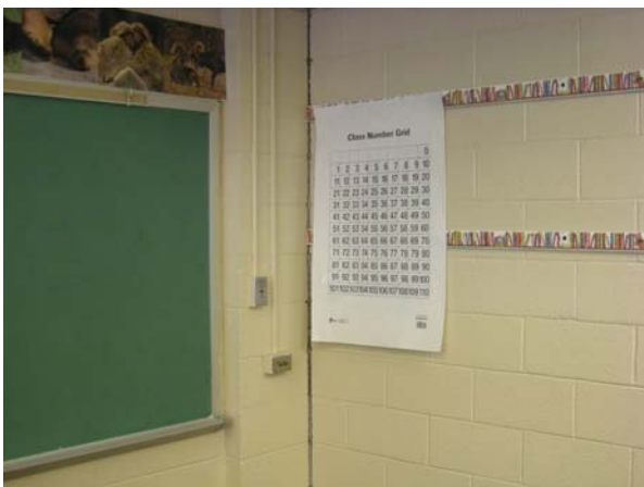
Separation of partition wall from interior wall
