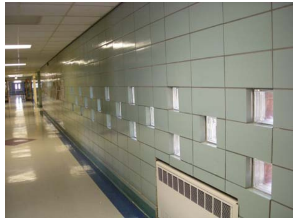
Lowest course in SGFT wall shifted
