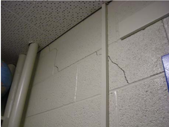
Cracking in CMU partition wall
