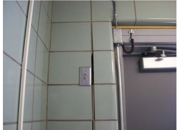
Cracking in SGFT wall
